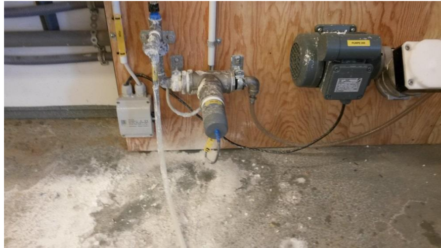
Figure 11.1: Operation leaks during the test period.
