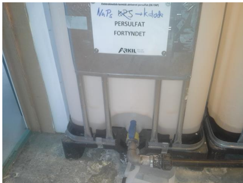
Figure 8.3: Connection of the buffer tank and the persulfate tank recycling content to CW.
